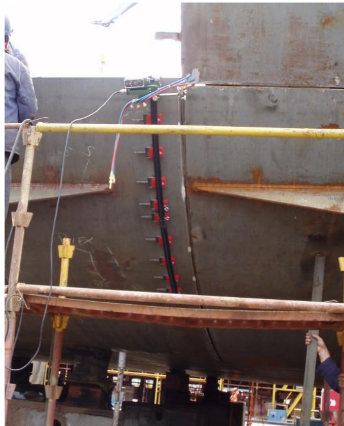
Welding preparation performed with 2D rail
