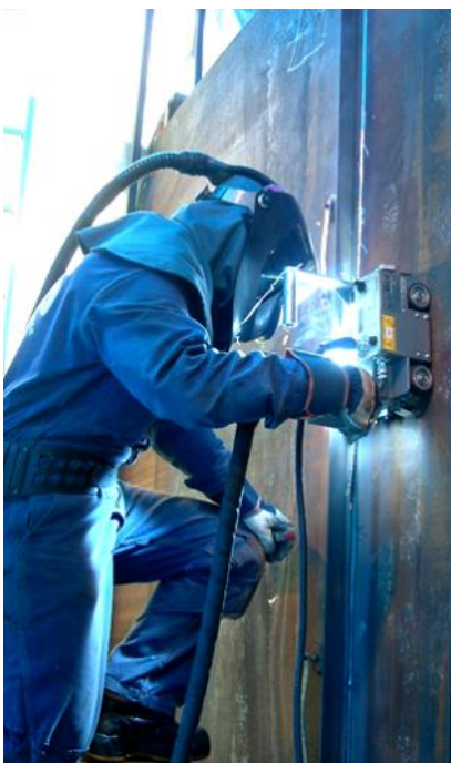
Vertical up butt welding using guide rail
